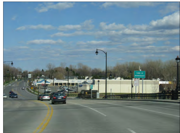
View from the east end of the O'Rourke Bridge along Pattonwood Drive toward Stutson Bridge plaza. Source: Clark Patterson Lee (2009)
