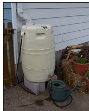
Residential rain barrel (upper), commercial rainwater cistern (lower) at Ryerson Woods Welcome Center in Riverwoods, IL. [Photo by Lake County, IL]
