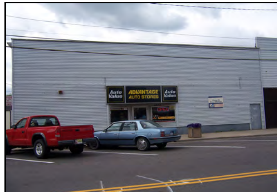
AVOID: Blank façade walls; discourage materials, inadequate windows, lack of symmetry or architectural details.
