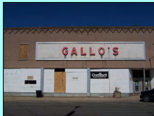
Low-cost or inconsistent building materials can transform well-made structure into eyesores.
