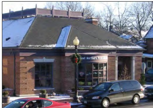
An example of an architecturally compatible roof screen used to conceal roof top mechanical equipment.
