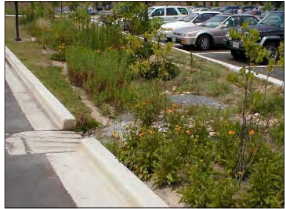
Rain garden in a parking lot in Monroe County, Indiana. [Photo by Monroe Co, IN]
