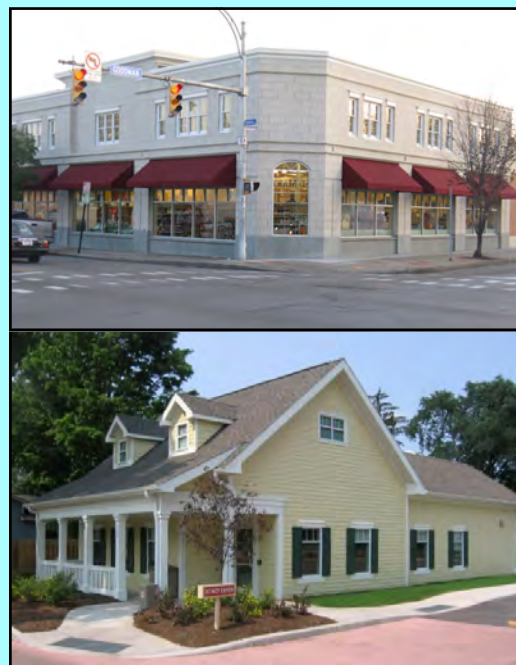
Above: RiteAid on Monroe Avenue has been designed so the building can be divided into smaller storefronts if vacated in the future. Bottom: Tim Hortons's building could be adapted to accommodate other uses.
