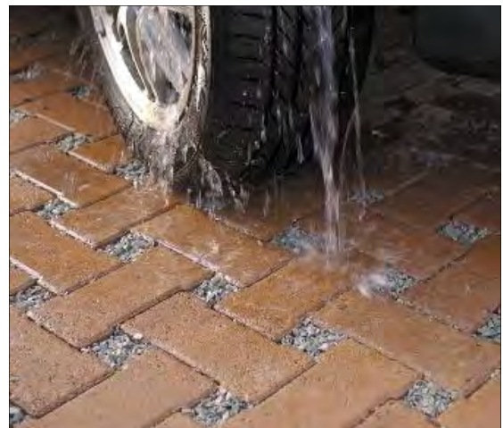
Pervious pavement as brick pavers. [Photo obtained from "mytorontohomeimprovement.com"]
