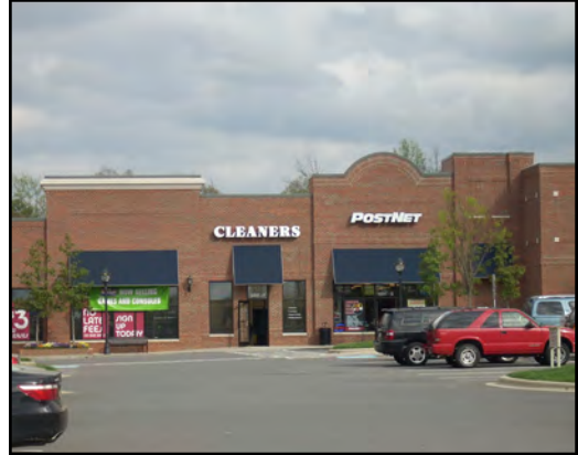
Lack of mass divisions or variation in material in the façade makes it difficult to see division of space at the pedestrian level.
